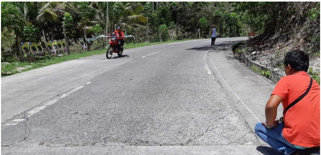
**FIGURE 22: SCALING OF CONCRETE SURFACE AT PACKAGE 1 (AWANG-NORTH UPI ROAD SECTION)**
