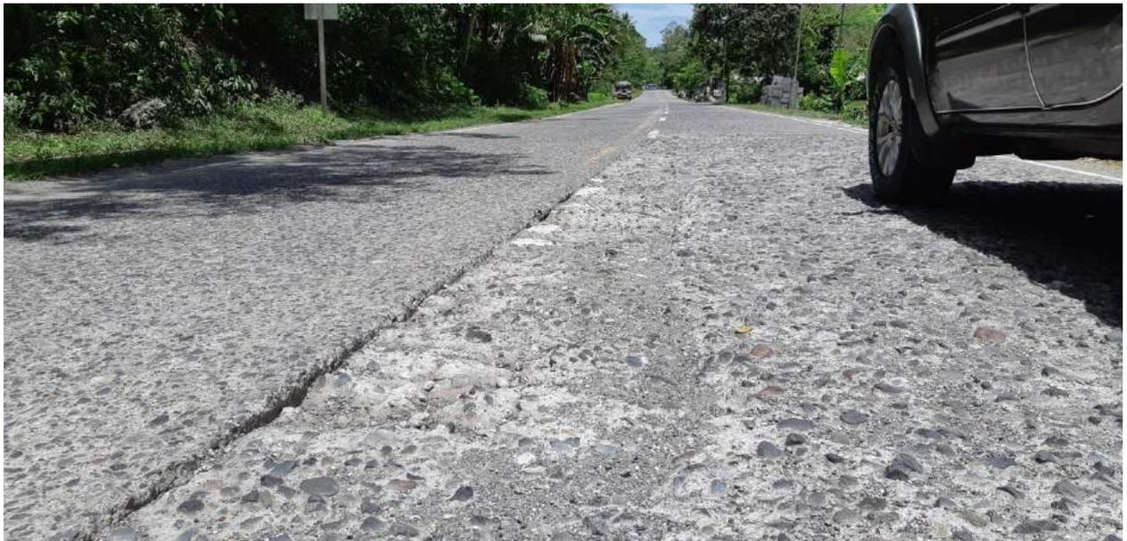
**FIGURE 24: SEVERE SCALING OF CONCRETE AT PACKAGE 2 (NORTH UPI - SOUTH UPI ROAD SECTION)**
