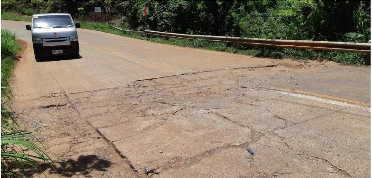
**FIGURE 23: SEVERE CRACKING AND DEPRESSION AT PACKAGE 2 (NORTH UPI-SOUTH UPI ROAD SECTION)**
