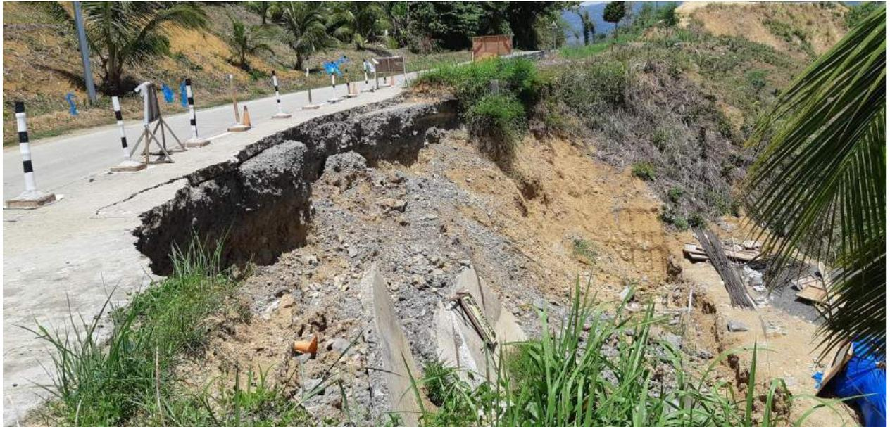
**FIGURE 25: ROAD SLIP AT PACKAGE 3 (LEBAK-KALAMANSIG ROAD SECTION)**
